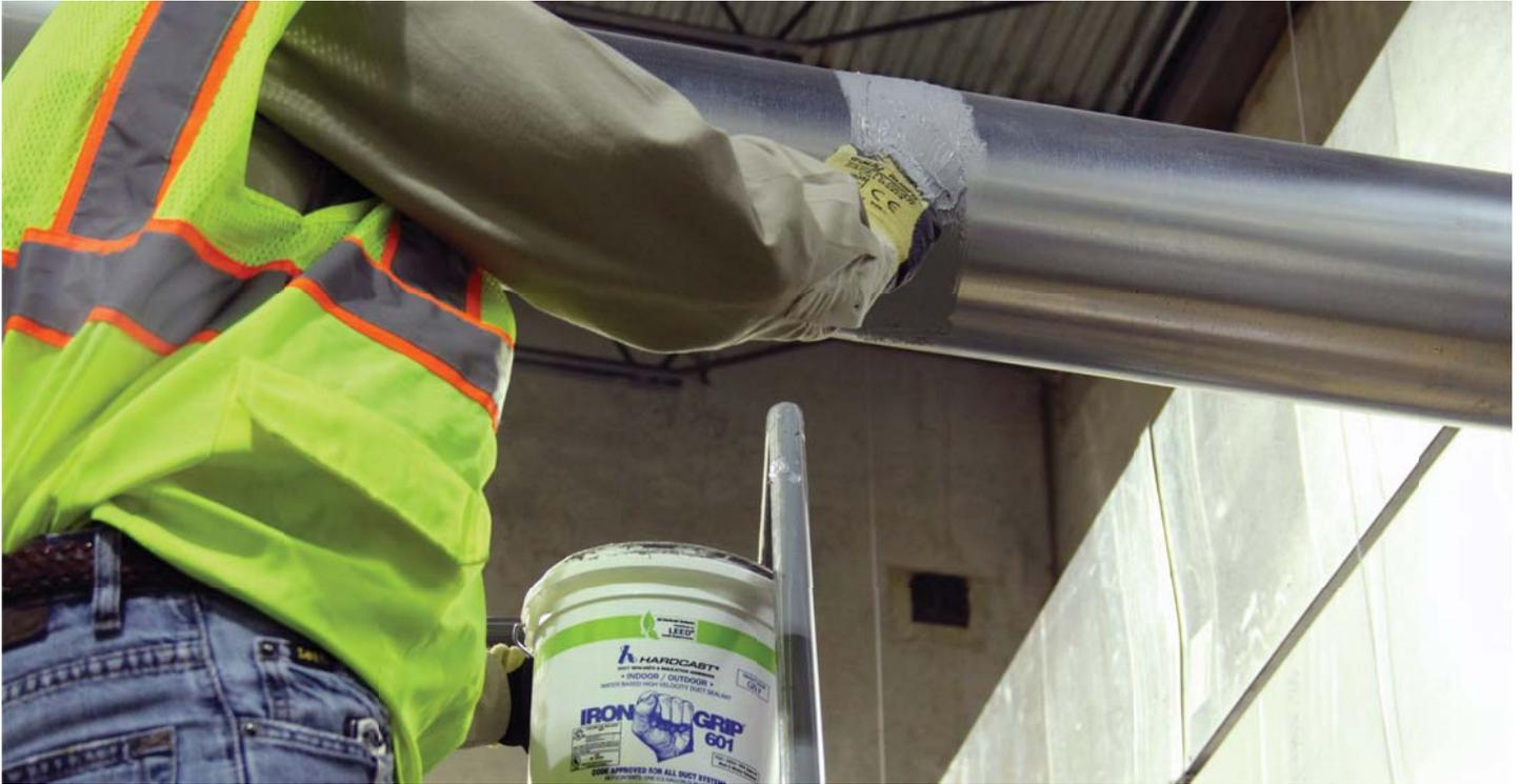
mastics sealants), brush-on sealants, sprayable sealants and coatings, and robotic duct-sealing devices — designed to boost the efficiency of HVAC equipment, usually focusing on keeping ductwork clean and leak-free.
