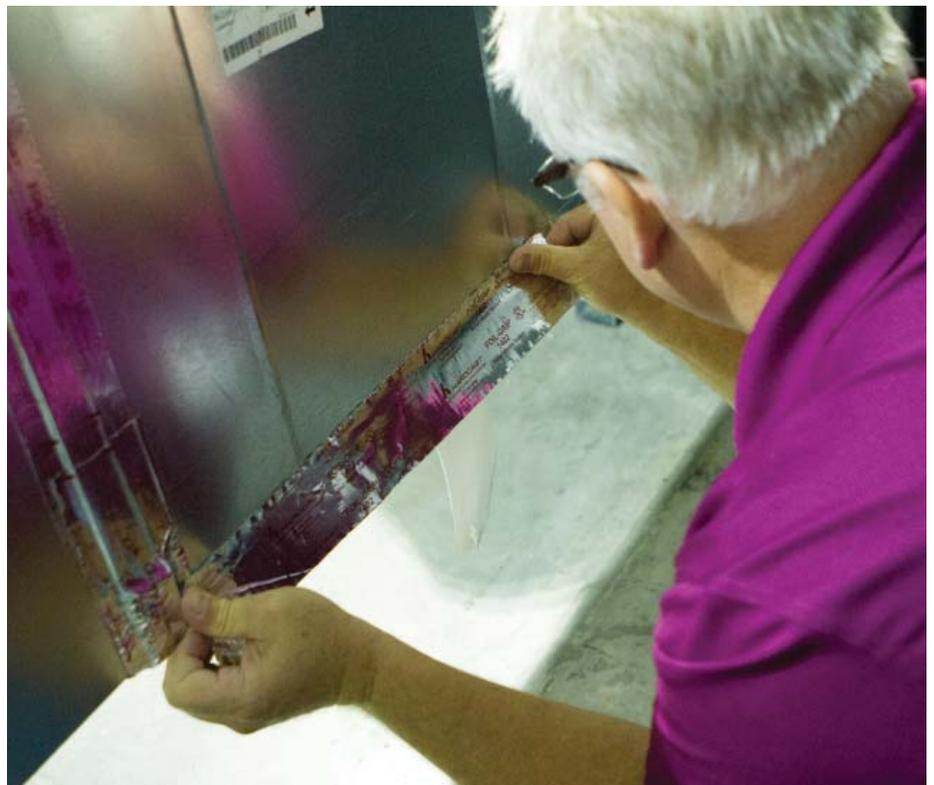
especially at the HVAC system's registers, air handlers and return-air vents, was responsible for 70 percent of the system's total reduction in air leakage. Manually applied sealants also had the shortest payback time — just over two years.
