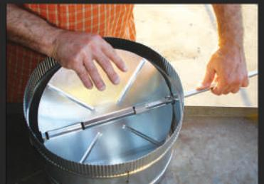
**3.** Spotweld or rivet the regulator in place, making sure the handle and blade are in corresponding positions
