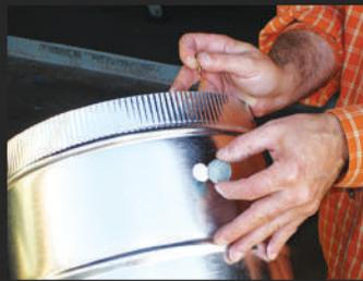
**2.** Holding the blade in position, pass the 3/8" square bar through the bushings and the channel in the blade
