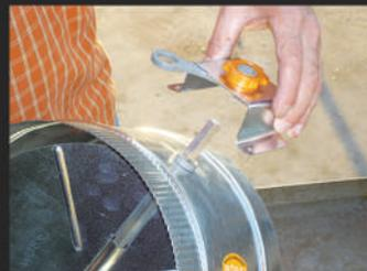
**4.** Center the blade and secure the system with a self-drilling screw
